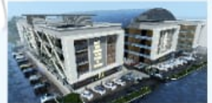
Mall & Shop Units etc
